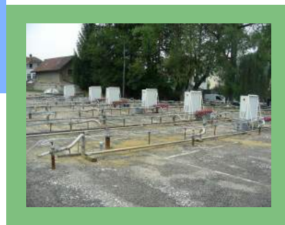
Assainissement in situ
