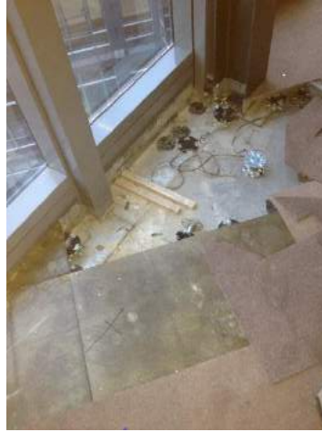
Faux-planchers Bureaux – Paris
