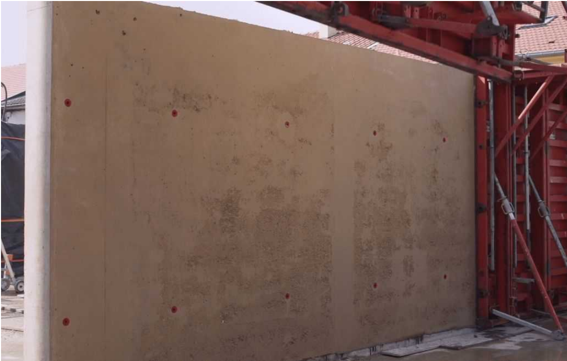
Poured earth, Saint-Clair-de-la-Tour, France
